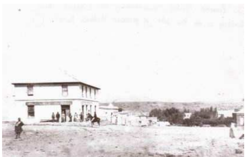
An early photo of Cradock taken from the upper corner of the Town Square. It shows the present Victoria hotel.
